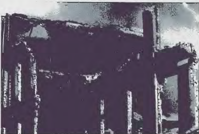
Cause: POOR EQUIPMENT MAINTENANCE
