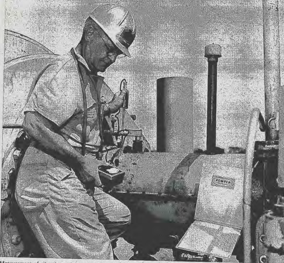
Measurement of vibration at inboard bearing of a steam turbine driving a high-speed centrifugal compressor.
