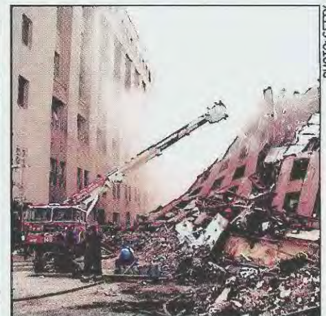
Firefighters spray water on the rubble of the World Trade Center on Sept. 12, 2001.
