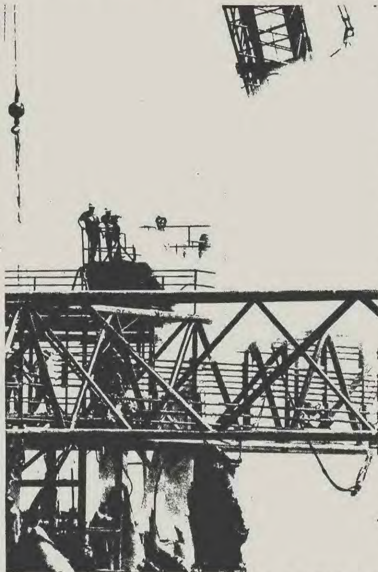
Red Adair's wild well control specialists sprayed the Shell Oil Co. Gulf of Mexico wells for five days after a 133-day fire and were not able to cap them until April 16. Two Shell employes injured when the fire began last Dec. 1 were fully covered for hospitalization and lost earnings through the company's self-insured workmen's compensation fund. Damage to the platform and equipment was covered by Lloyd's of London. Four employes of Storm Drilling Co., Houston, who were killed were covered by life insurance placed through Adams & Porter. Damage to two of Storm's drilling rigs and related equipment was covered by insurance split between the domestic and foreign markets.
