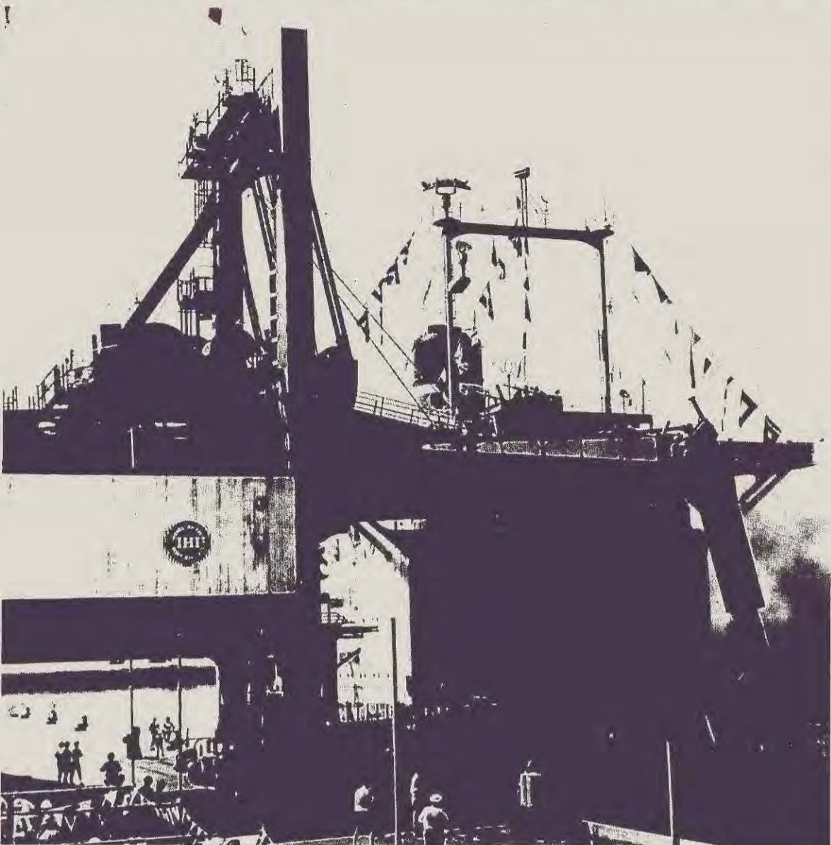
One of the world's largest ship loaders can transfer 8,000 tons of ore an hour to giant cargo vessels. Here, the ship Osumi Maru is being loaded at Port Hedland, marking the first commercial shipment of Mt. Newman ore to Japan on April 1, 1969.
