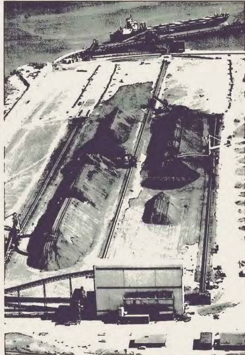
This aerial view shows ore-loading facilities of the Mt. Newman iron ore project. The pier is being extended some 1,000 feet to accommodate two ships or a larger vessel.
