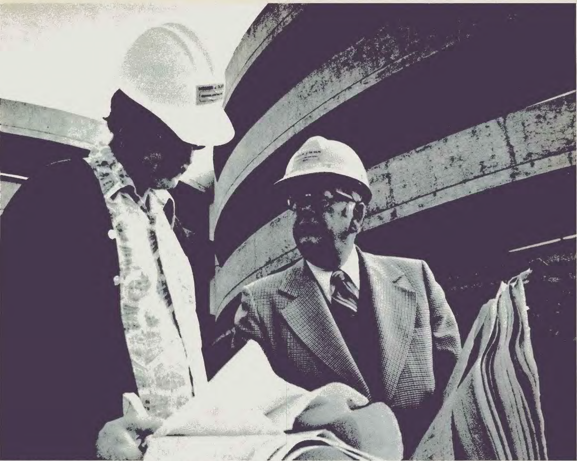
The better the plan, the better the work. Here, Homer J. Olsen, right, and project manager, Stan Summers, confer on the site of a recent Bay area job.
