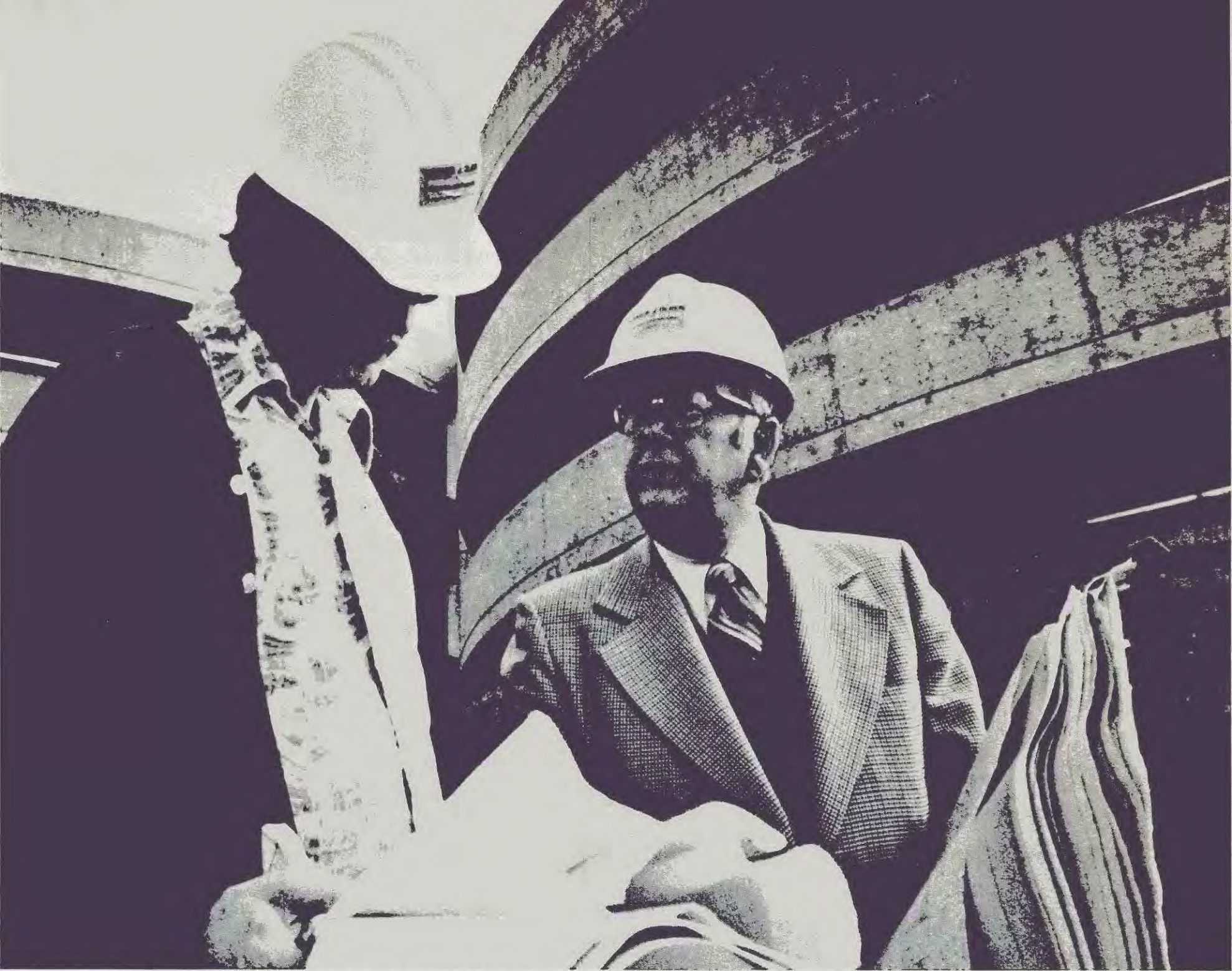
The better the plan, the better the work. Here, Homer J. Olsen, right, and project manager, Stan Summers, confer on the site of a recent Bay area job.
