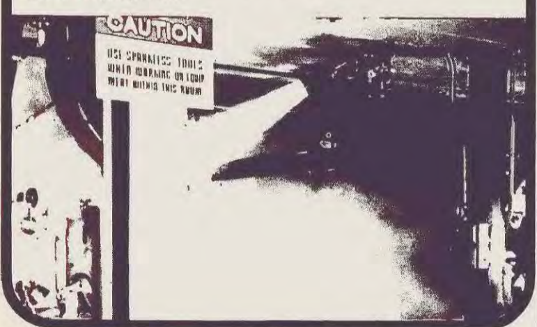
High-pressure Cardox Carbon Dioxide System protects against fire in "White" Room at Charles Bruning Company, Division of A-M Corporation, Mount Prospect, Illinois.
