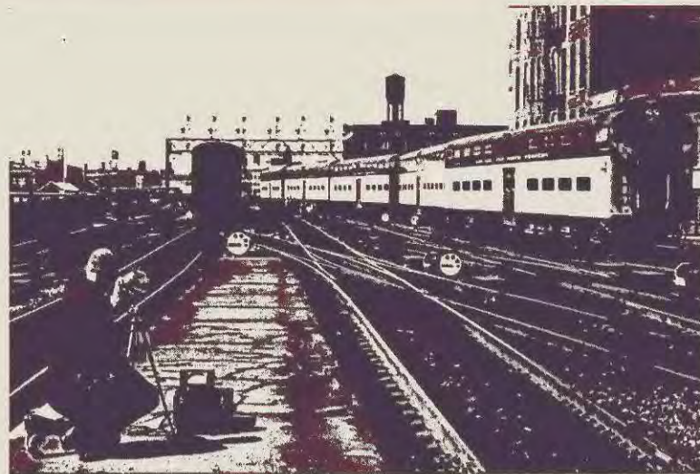
The use of portable radar units to check the speed of trains is one of the many audits of the Chicago & Northwestern Railway Co.'s new safety program.
