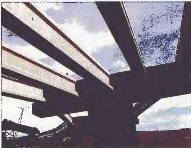
To provide workers' comp and liability coverage for a construction project that employs dozens of trades takes flexibility and resourcefulness. It takes a company like Argonaut.
