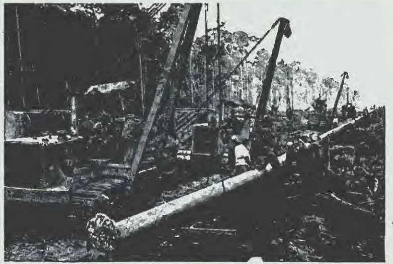
Bechtel employes laying pipeline in Indonesia.
