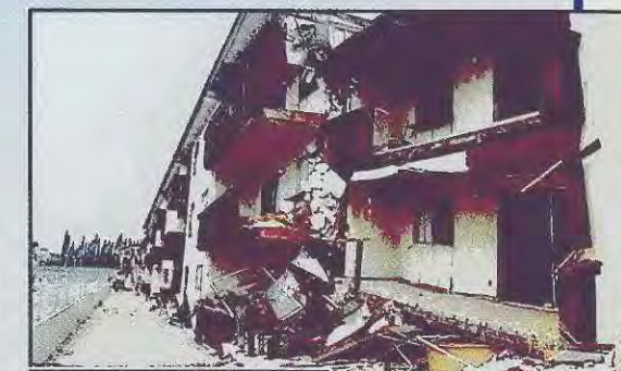
The collapse of buildings such as the Northridge Meadows apartment complex in the 1994 earthquake has led to closer scrutiny of the components used in construction.
