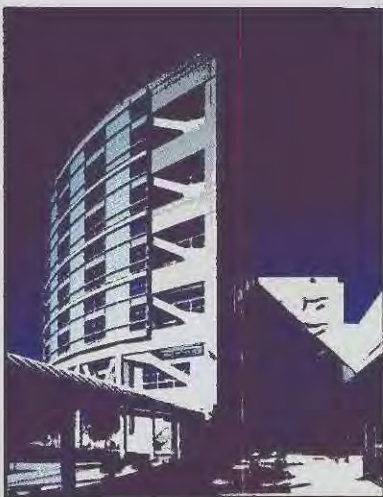
PHOTO: JOHN LINDEN/ESTO PHOTOGRAPHICS The new Arrowhead Regional Medical Center in San Bernardino, Calif., was designed to withstand quakes.
