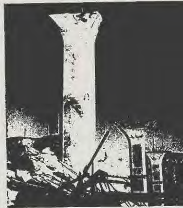
1971 earthquake demolished expressways in the Los Angeles area.
