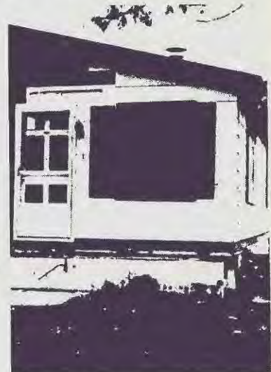
This modular home in Love Canal was split for moving it out of the contaminated area.
