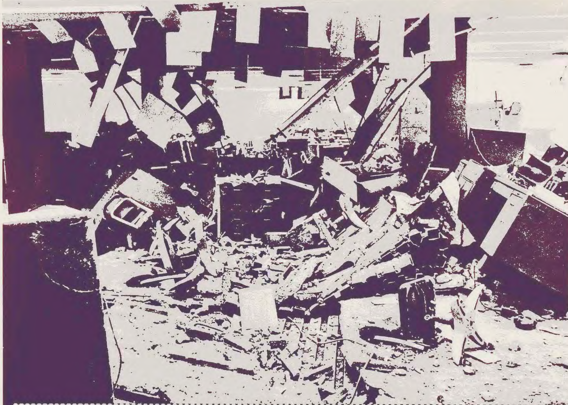
(AP) ALBANY, N.Y., ---BUSINESS UPSET---This was the scene yesterday in the office of a local realtor after a boiler exploded in the room below. Floor and roof collapsed, destroying office equipment. There were no occupants in the building at the time of the accident. (AP) (bfw638594/8571kp) 1967
