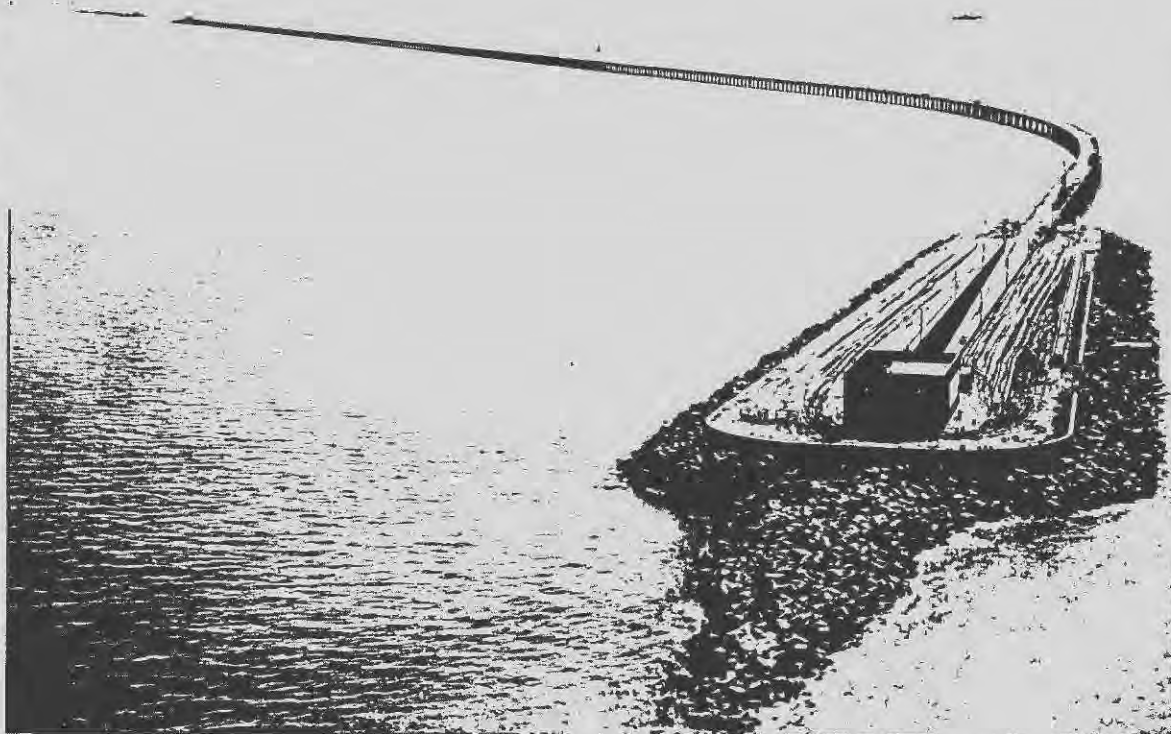
Over and under the seas is the course of the Chesapeake Bay Bridge Tunnel which has a total length of 23 miles, with 17.6 across the water. A diesel boat "Surveyor" keeps a constant check on the bottom and quickly makes necessary repairs before serious problems develop.
