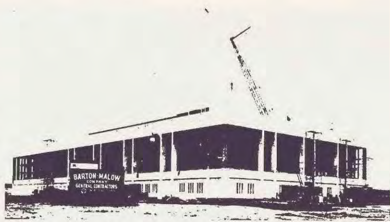
General contractor for the Henry Ford Centennial Library in Dearborn, Mich., Barton-Malow Co. holds that construction workers, who by their nature are "show-offs," should be educated in safety rather than be ordered to follow safety procedures.
