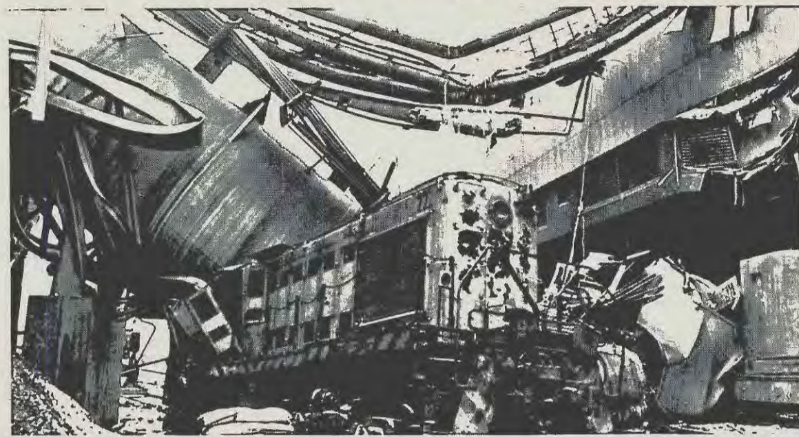
United States Steel Corp.'s basic oxygen furnace shop in Gary, Ind., was the scene of tragedy as three workers were killed and five others injured in the collapse of an air pollution control pipe. The fallen pipe, 16 feet in diameter, caused damage estimated at $3.7 million and forced U. S. Steel to shut the plant down. Officials of U. S. Steel said the company is self-insured for workmen's compensation, property damage and business interruption. -Gary Post-Tribune
