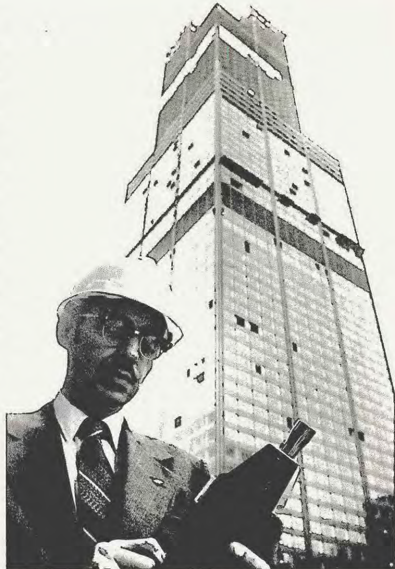
OSHA inspector Bill Kafka takes a reading from his noise meter in front of the Sears Tower construction project in Chicago. Random checks comprise about one-half of Illinois' OSHA inspections.
