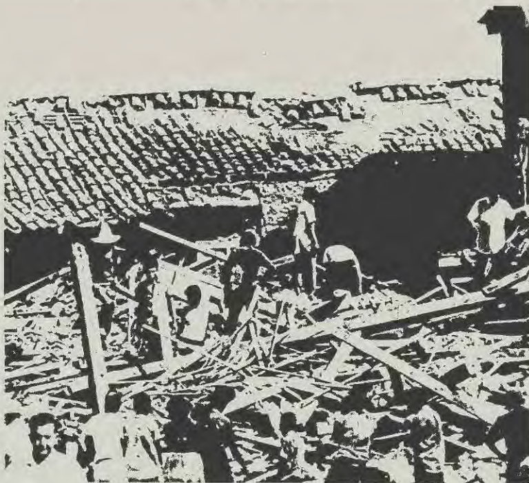
Damage to Managua, Nicaragua, might be as high as an estimated $2 billion, following an earthquake there Dec. 23. —Wide World photo
