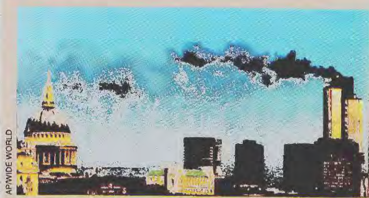
A fire at NatWest Tower in London's financial district last week was quickly brought under control. Damage from the rooftop blaze, which is insured, did not appear to be extensive.
