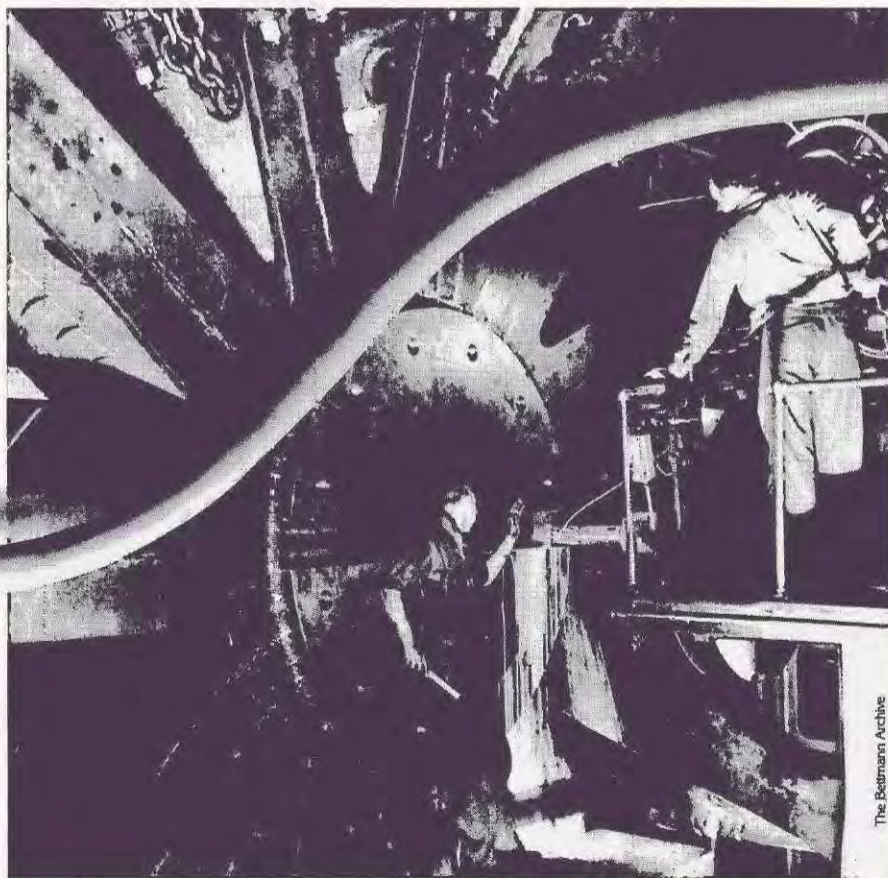
Part of the huge rotor for the waterwheel generator used in the Tennessee Valley Water Plant
