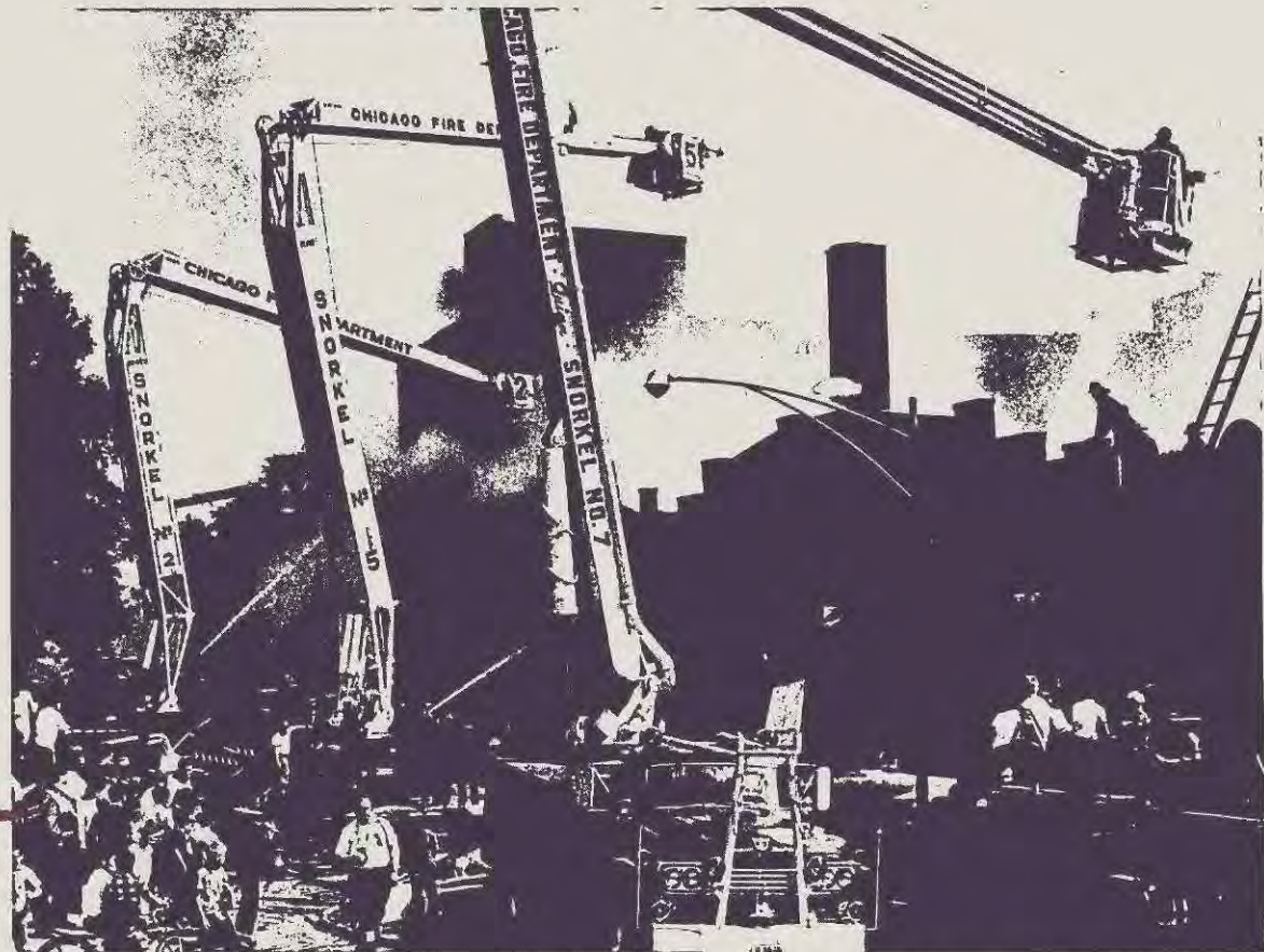
A blaze that began while a new mixture was tested at the Wellco Chemical Co., Chicago, did $100,000 damage to the plant and to the neighboring Apco Plating Co., when the roofs of both buildings collapsed. An estimated 50 employees escaped without injury. More information on U.S. fire losses since 1947 is presented on page 12. Chicago Sun Times, Joe Kordick.
