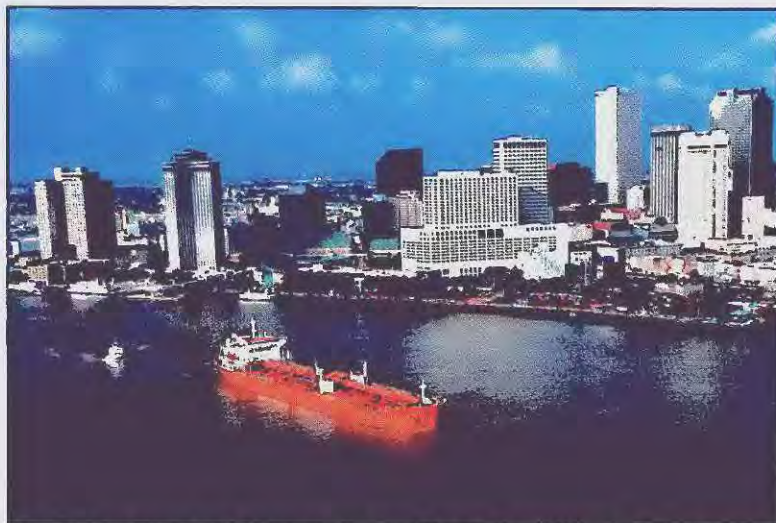
New Orleans property owners worry that low water pressure, already below average before Hurricane Katrina, is jeopardizing fire safety systems.
