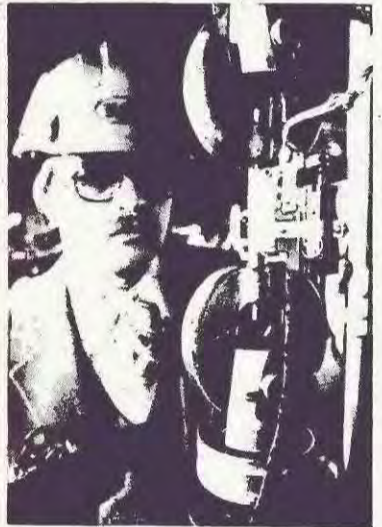
Photo: Hartford Steam Boiler
