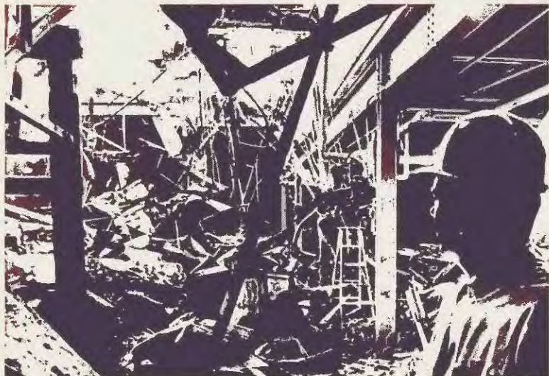
An unidentified workman in the Utica-Mohawk textile plant in Clemson, S. C., investigates the aftermath of an explosion that killed three in this cotton textile plant, a subsidiary of J. P. Stevens & Co., New York. A Stevens spokesman said that loss will exceed $1,000,000. Carriers include the Factory Insurance Assn. and Liberty Mutual. An 80-foot long drier, which exploded, was "equipped with all the safety devices known to man," the spokesman said. Wide World photo
