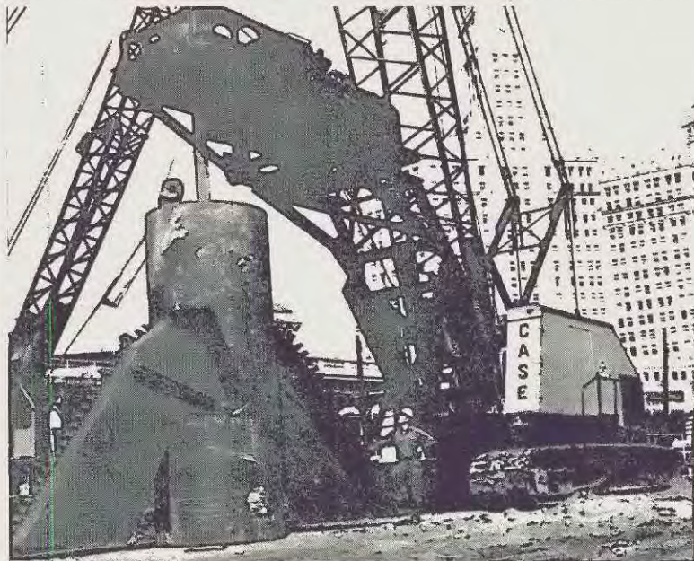
The teeth on the sides of this belling bucket, and similar pieces of machinery, were discovered to be one of the main causes of eye injuries for Case International Co. workers. Use of the current-costing program developed by Employers Insurance of Wausau revealed the problem area and enabled Case to work out three safety steps that have reduced the number of such accidents substantially.
