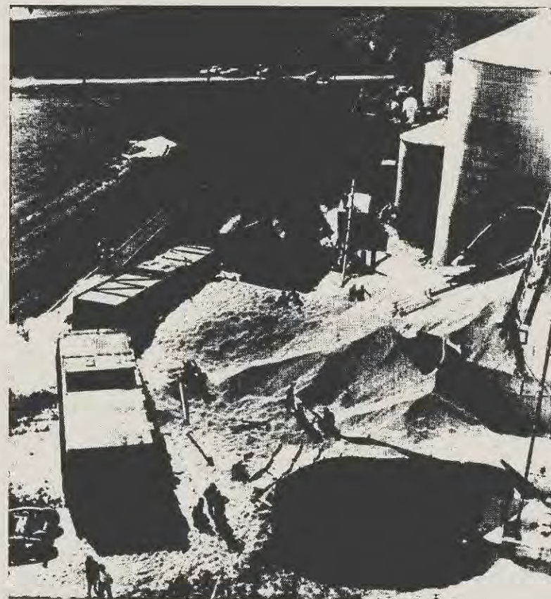
The Kruse Grain Co., Cleves, Ia., suffered an uninsured loss in this mishap that was estimated more than $135,000. Three nearby railroad boxcars were knocked over when about 70,000 bushels of corn burst from a storage bin. A structural weakness in the bin was the indicated cause of the loss. After friends and neighbors helped clean up the corn, Ernie Kruse, manager, said he is thinking of making a claim against the manufacturer of the bin. The clean-up operation took two days to complete. —Wide World photo
