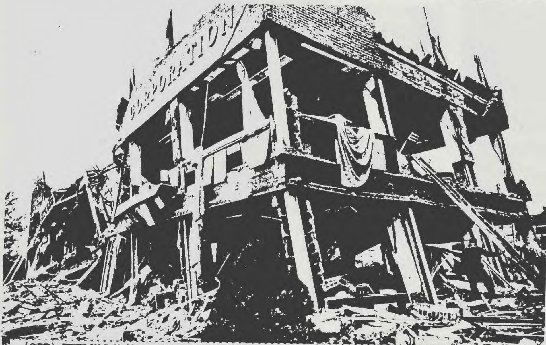
(AP) NEW YORK, N.Y.---EXPLOSION SITE---The remaining walls and rubble of the executive office building of a major appliance manufacturing firm ripped apart during an explosion are shown above. Fortunately the accident occurred on a Sunday when employees were at home. (AP) (abk857/4251kp) 1968.
