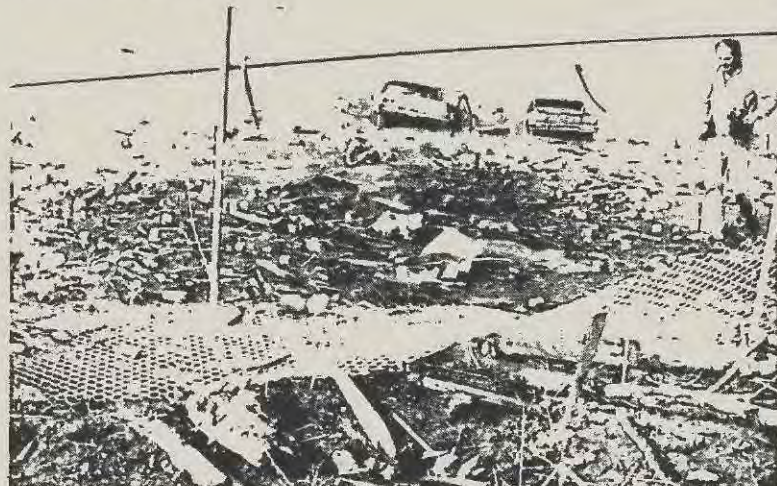
A fireworks holocaust obliterated 16 of 18 structures comprising the Melrose Fireworks Display Co. Property damage estimates are still pending on the effects of explosions felt over a 10-mile radius.
