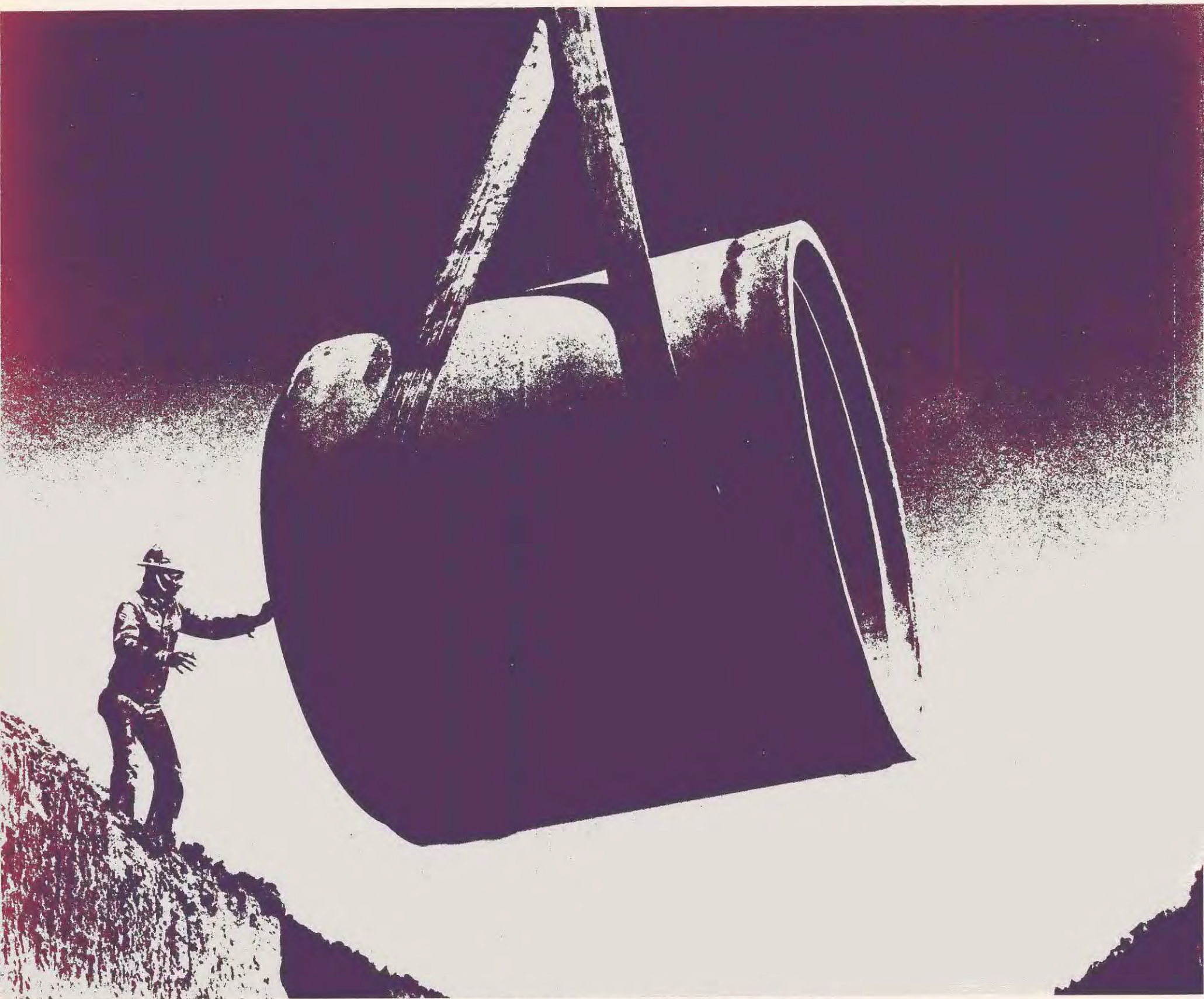
Laying 20-ton pipe at the Foothills Treatment Plant in Denver, Colorado.
