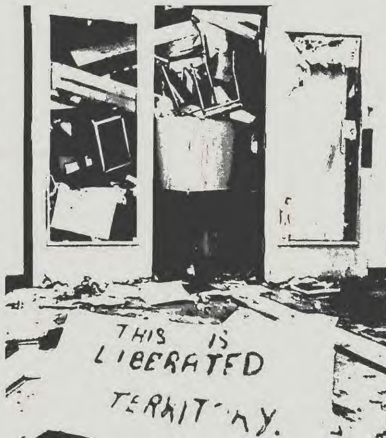
Insurance covered a major share of a loss estimated at $2,300,000 at Sir William George University, Montreal, where students rioted and barricaded themselves in this computer center. Protesters almost totally destroyed the university's EDP installation. —Wide World photo
