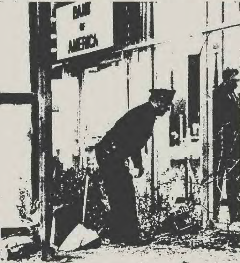
The Kaiser Center Bank of America branch, Oakland, Cal., suffered approximately $10,000 damage when a bomb exploded against the pillar at the left. The bombing was one of 30 that have hit various branches of the bank in the past 14 months. —Wide World photo
