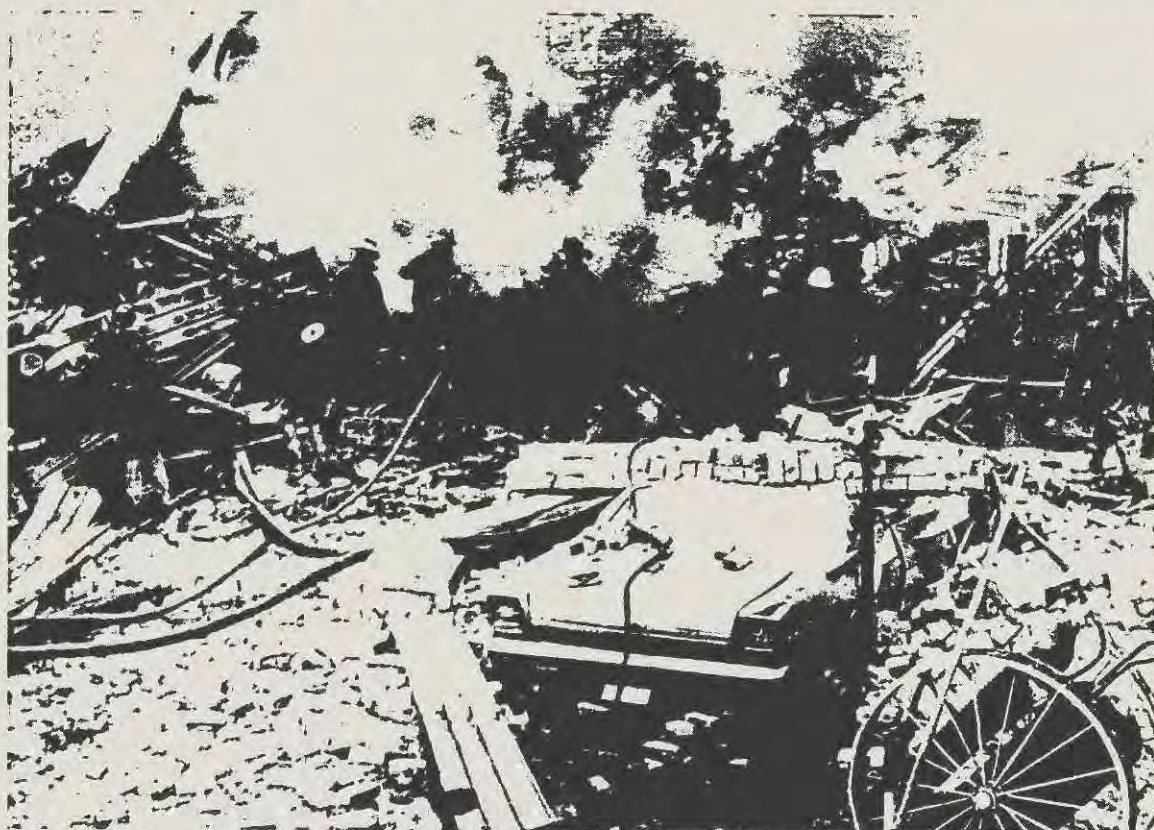
The Chicago Transit Authority, a publicly operated system, suffered a bus garage explosion-fire that caused $500,000 estimated damages and injured 88, six seriously. Business Insurance learned the CTA is self-insured for $300,000 of the fire damage but the remainder is covered by a $3 million-limit fire insurance policy with Lloyd's. In addition, Lloyd's provides public liability policy for a undisclosed limit after a $1.5 million deductible. Wide World photo
