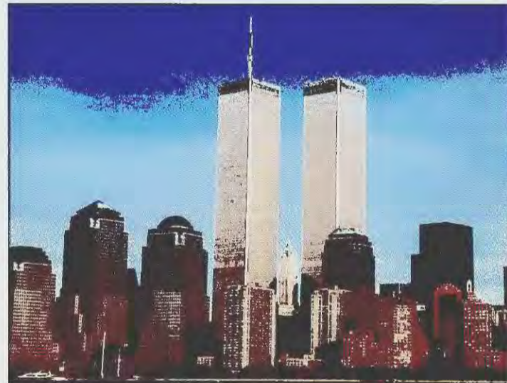
ABM Industries Inc., a janitorial services contractor for the World Trade Center, could recover more than $127 million for business interruption losses stemming from the destruction of the buildings.
