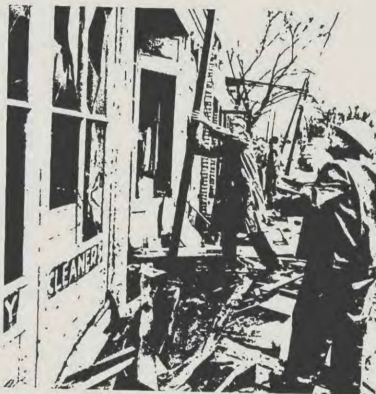
Tornadoes did an estimated $2,000,000 damage in Greenwood, Ark. Residents remove debris after a late April tornado struck the town of 2,000, leveling most of the business buildings on the city square. Insured losses from tornadoes and hail in five other states are estimated at $6,500,000. The states include Indiana, Kentucky, Michigan, Ohio and Tennessee.
