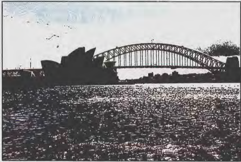
Two tunnels now under construction beneath Sydney Harbor, site of the Sydney Opera House, are expected to be completed in 1992.
