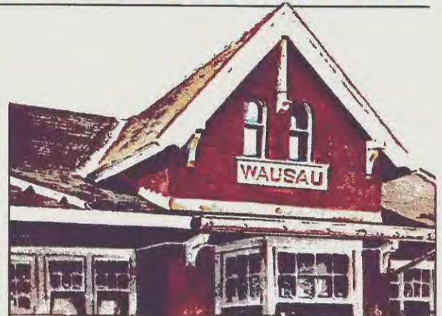
Robert Johansen chose to capture the charm of our depot in one architectural detail.
