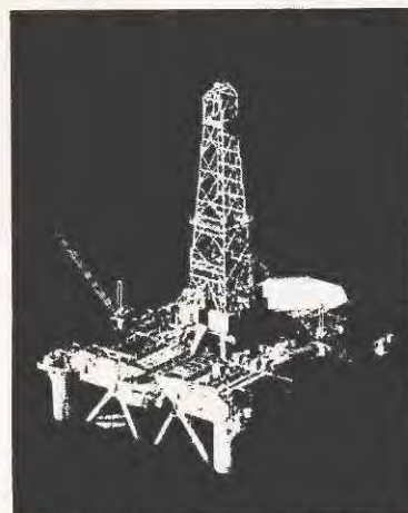
Offshore drilling rigs are an example of some of the "tough risks" covered by Pru Re.
