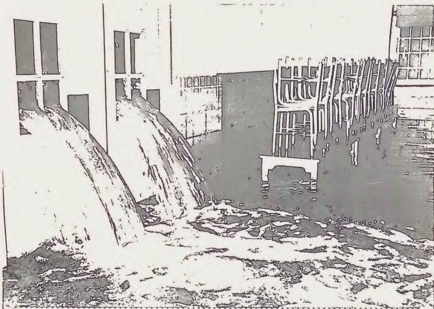
( ) ,CONN.---LUNCH WILL BE LATE---A primary water main burst early yesterday morning in an employe cafeteria basement sending cooks and some early morning coffee drinkers scurrying for safety. Business went on as usual but the cafeteria was closed until further notice. ( ) 1kp0 1968.
