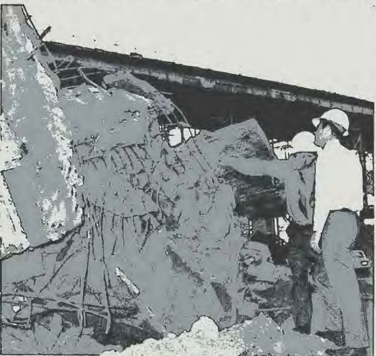
Officials of the California state highway department inspect damage caused by the 1971 San Fernando earthquake.
