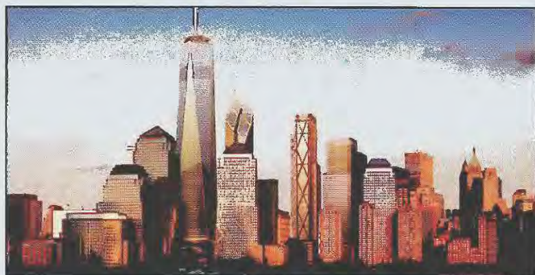
The proposed rebuilding of the World Trade Center may not proceed exactly as leaseholder Silverstein had planned after a federal judge ruled the leaseholder can only recover the cost of the towers as they stood before Sept. 11, 2001.
