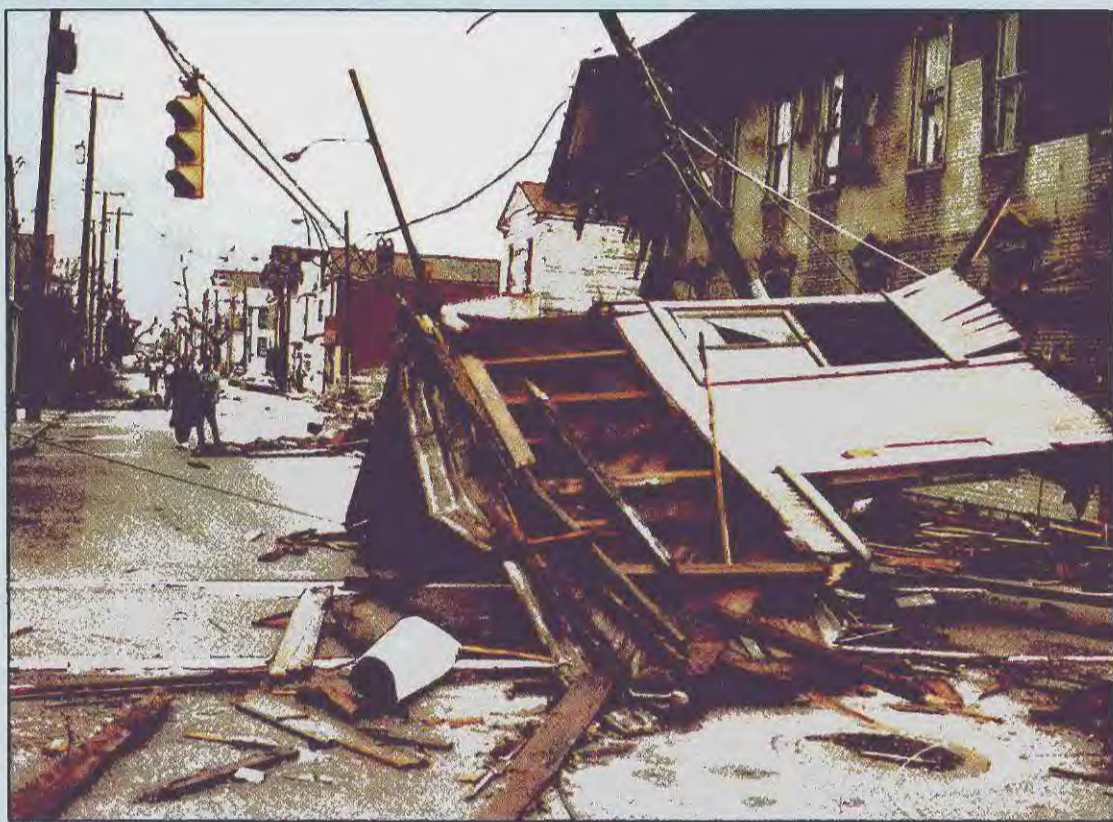
Hurricane Hugo damaged an estimated 300,000 buildings in Charleston, S.C., alone.
