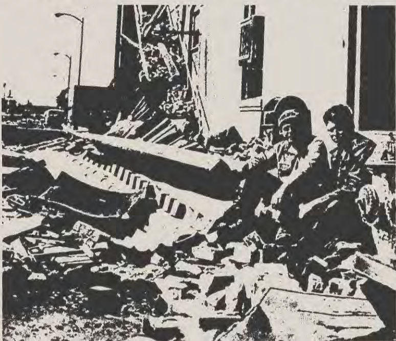
A series of earthquakes jarred Sonoma County, California, and it is now estimated the city of Santa Rosa suffered about $5 million in damage. The Santa Rosa Memorial Hospital was hit with $100,000; 40 homes were damaged beyond repair and 200 were seriously damaged. Because of normal exclusions for earthquake damage, most businesses and individuals are uninsured. The city will have to pay for most of the damages out of self-insurance. —Wide World photo
