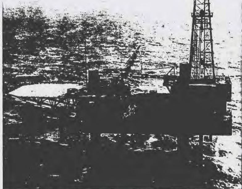
Despite the Coast Guard's contention that oil spill liability is not unlimited, risk managers and insurers aren't so sure.
