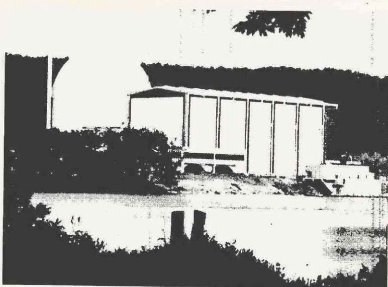
The nuclear power plant of the Connecticut Yankee Atomic Power Co.
