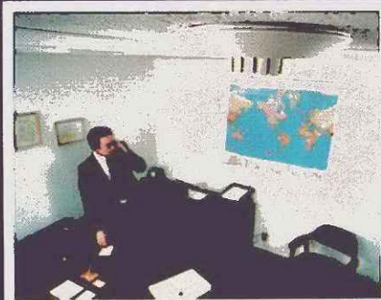
Early warning is provided by ionization smoke detectors, which sense invisible products of combustion. May be coupled with thermal or photo-electric detectors.
