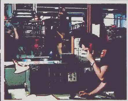
Fire alarm signals are immediately transmitted to municipal fire department.
