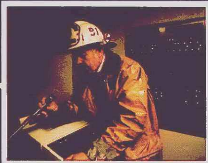
Fire command center gives battalion chief up-to-the-minute status information. Provides audio communications equipment and remote control of fan systems.
