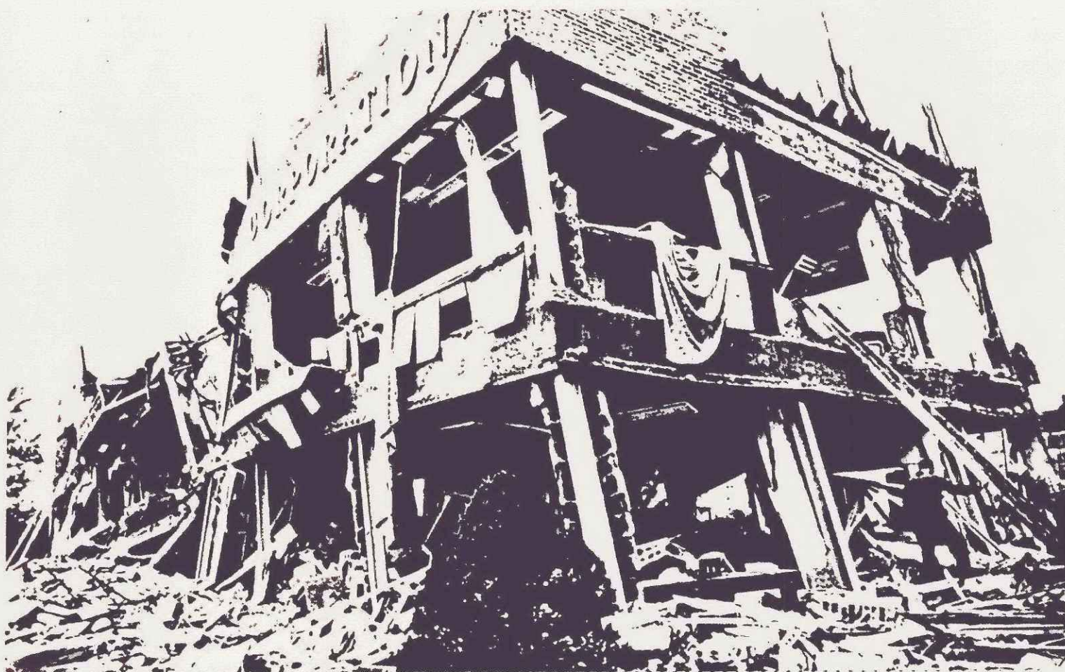
( ) N.Y.---EXPLOSION SITE---The remaining walls and rubble of the executive office building of a major appliance manufacturing firm ripped apart during an explosion are shown above. Fortunately the accident occurred on a Sunday when employees were at home. (abk857/4251kp) 1968.
