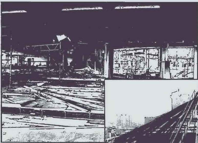
Flames and temperatures of about 1,800 degrees Fahrenheit gutted the building, destroying escalators and burning through the top of the atrium.
