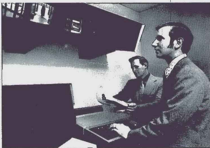
Clifford E. Evans, Security Director, and Lew Handeland, Building Engineer, review how Alpha 3000 responds instantly, automatically to emergencies. System is U.L. approved for Class A fire protection.
