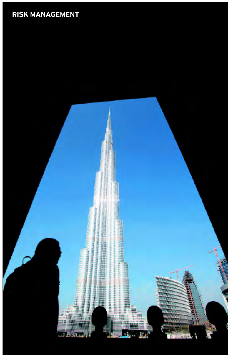
One view of the Burj Khalifa, the world's tallest building, which officially opened in Dubai, United Arab Emirates, last week.
