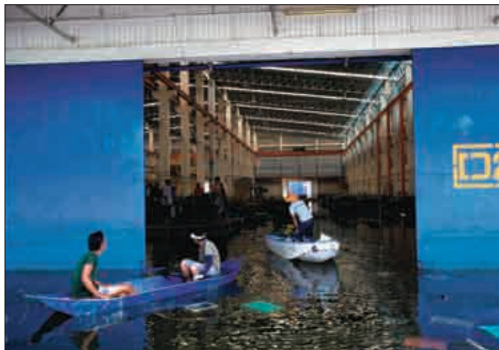
Facilities at an industrial park near Ayutthaya, Thailand, were inundated last year. Flooding in Thailand has caused billions of dollars in losses.
