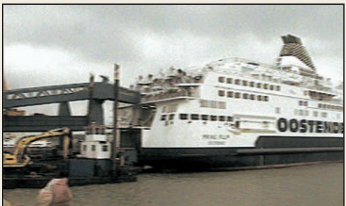
Two Swedish firms failed to pay fines in England stemming from the collapse of this walkway at the port of Ramsgate.
