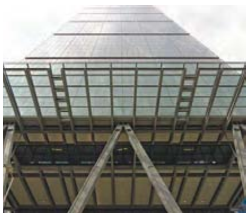
Three huge bolts plunged to the ground from the recently opened 47-story Leadenhall Building in London.
