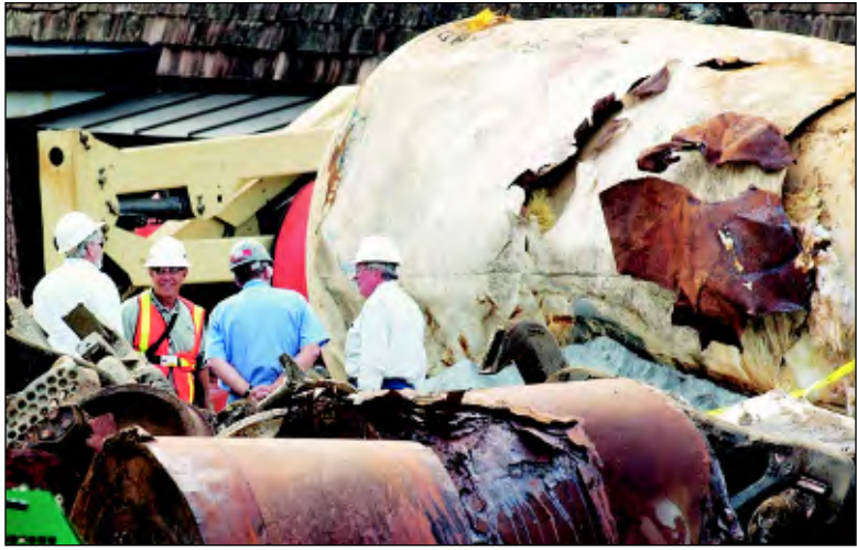
Contract workers for Norfolk Southern Railway Co. are surrounded by wreckage from a 2005 derailment that released deadly chlorine gas, killing nine people.
